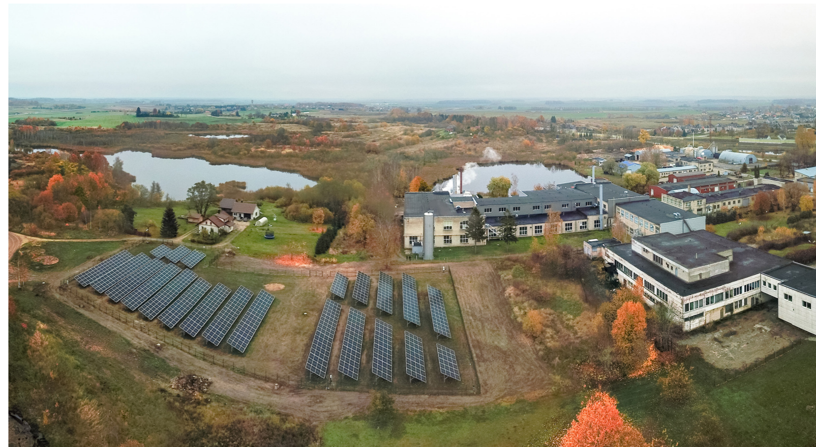
In November 2020, Gabriel's part-owned dyehouse, Scandye, established a solar cell park with a capacity corresponding to 17% of the dyehouse's annual energy consumption.
